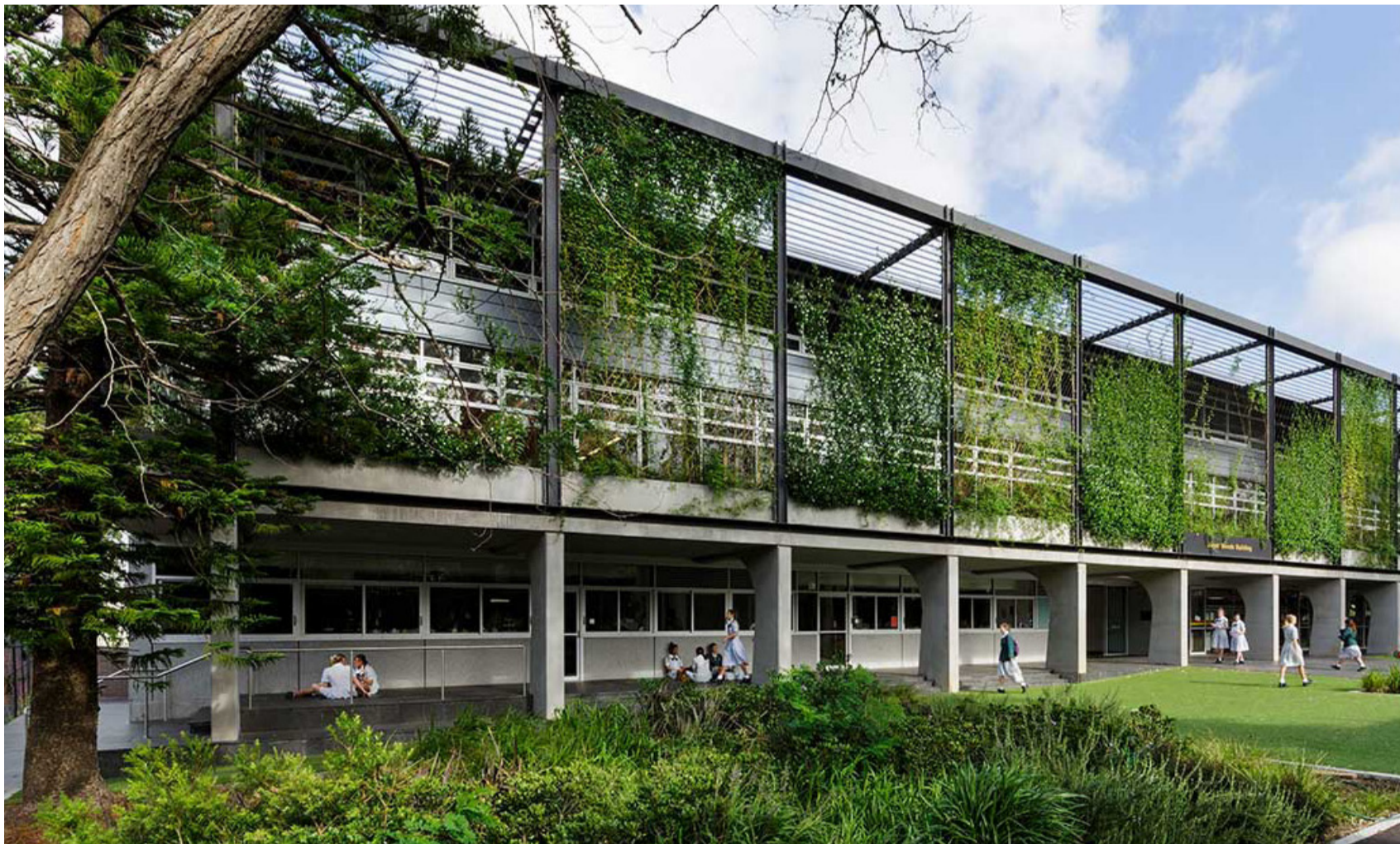
Stainless steel cable/mesh facade planter with social space beneath
