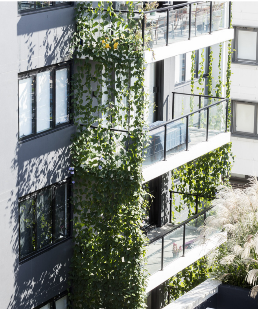
Steel cable / mesh enable planting to climb vertically up facade
